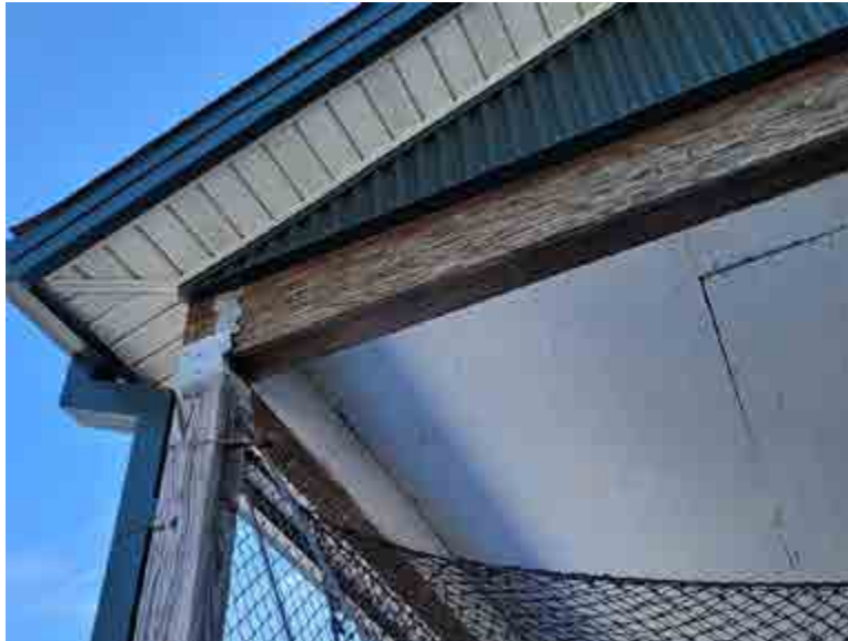
Weathered exposed wood framing at clubhouses.
