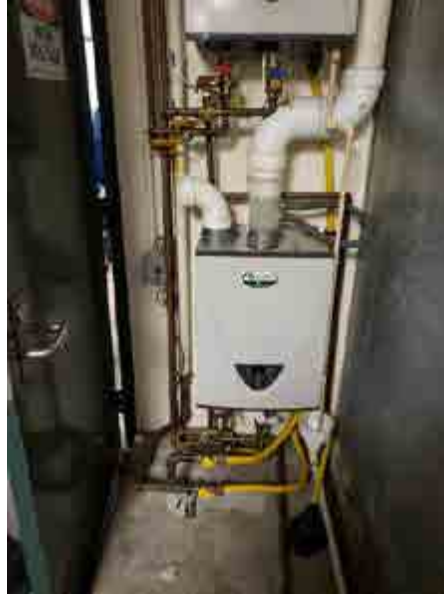
(2) Gas fired tankless water heaters serve the Commissary.
