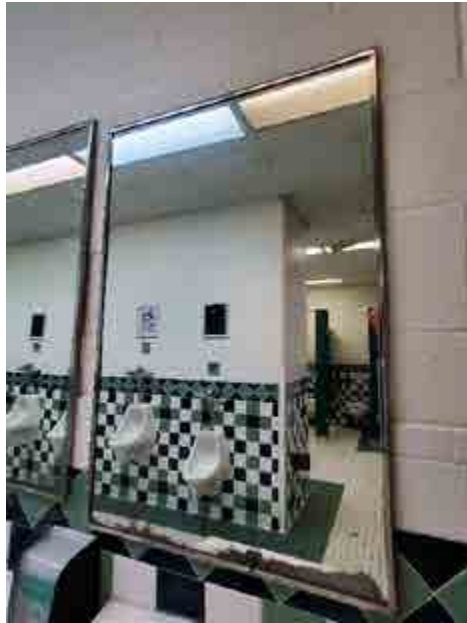
ASCI-12 Mirror delamination
