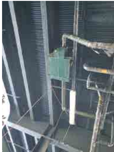
50 GPM Grease Interceptor at underside of structure serving the Buffet Kitchen above.
