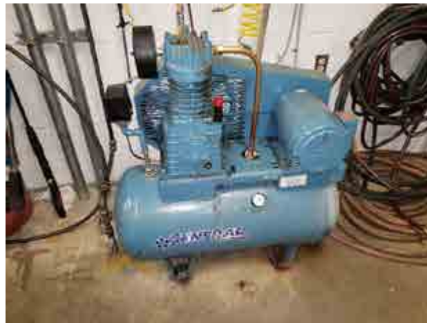
Dry Sprinkler System Air Compressor at Main Mechanical Room
