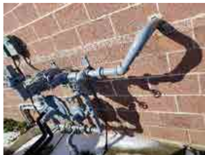
(2 PSI) Natural Gas Service Meter Assembly at Visiting Team Clubhouse
