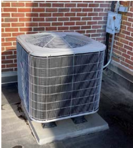
(15) Split System Air Conditioning Unit (AC-X)
