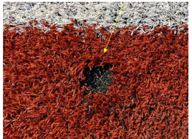
RUBBER BASE PLUG FOR 60' BASES. TODD WILL INSTALL TURF & INFILL ON TOP OF THE PLUGS PRIOR TO THE MiLB SEASON.
