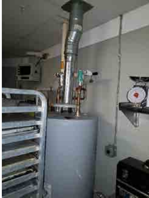
A gas fired 74-gallon storage tank type serves the Buffet.
