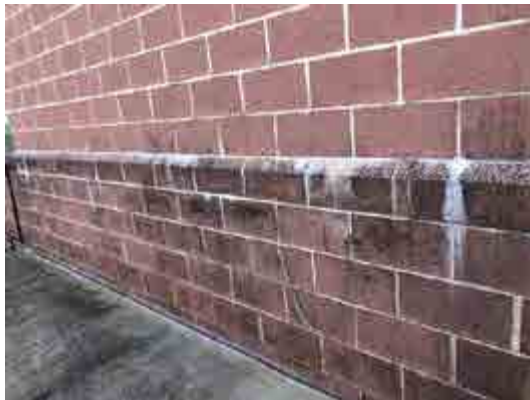
AHCE-1 Exterior CMU Wall Water Table
