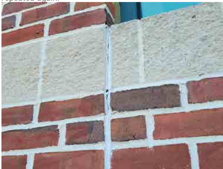
Failed contraction/control joint in brick veneer.
