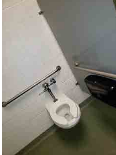
Manual flush valve Urinal and Water Closet at Home Team Clubhouse
