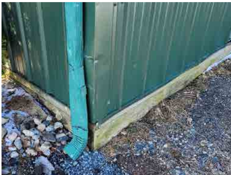
Deterioration of dimensional lumber curbs at storage buildings.
