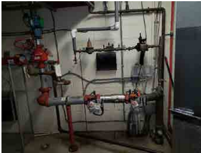
Picnic Bar Combined Fire and domestic water meter and backflow preventers
