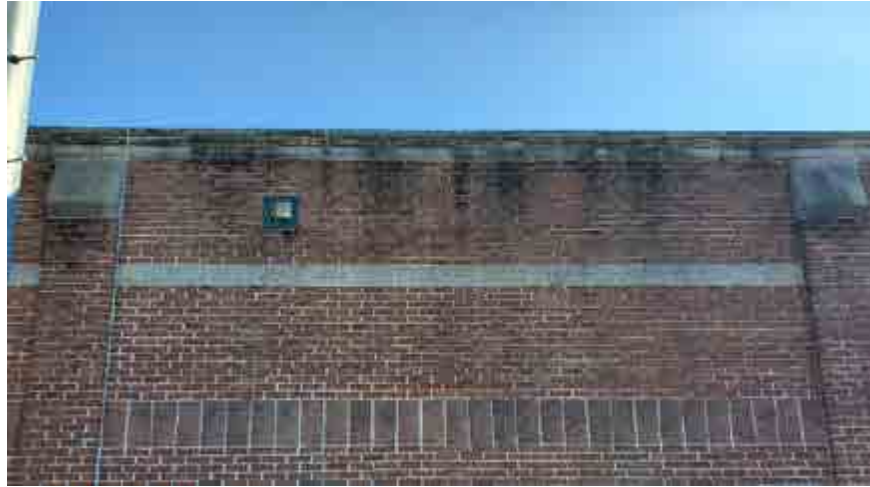
ASE-7 Masonry Parapet Caps
