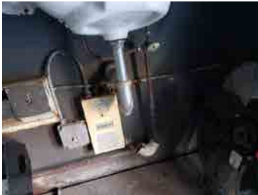
Electric Point of Use water heaters serve each Dugout
