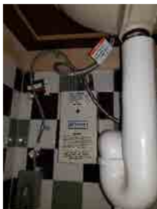
(12) Electric Point of Use water heaters are located below each lavatory and countertop sink to serve the Suites.
