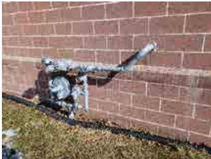
(2 PSI) Natural Gas Service Meter Assembly at Home Team Clubhouse
