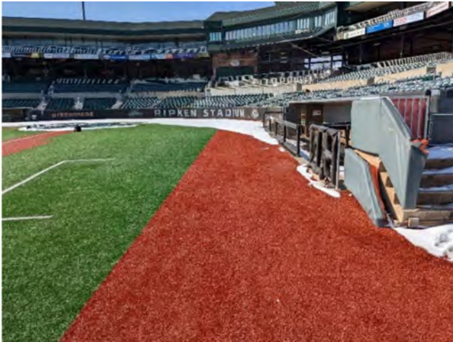
WARNING TRACK IN FRONT OF DUGOUTS DOES NOT MEET 15' MINIMUM WIDTH REQUIREMENT. WARNING TRACK DOES NOT PROVIDE TACTILE DIFFERENCE.
