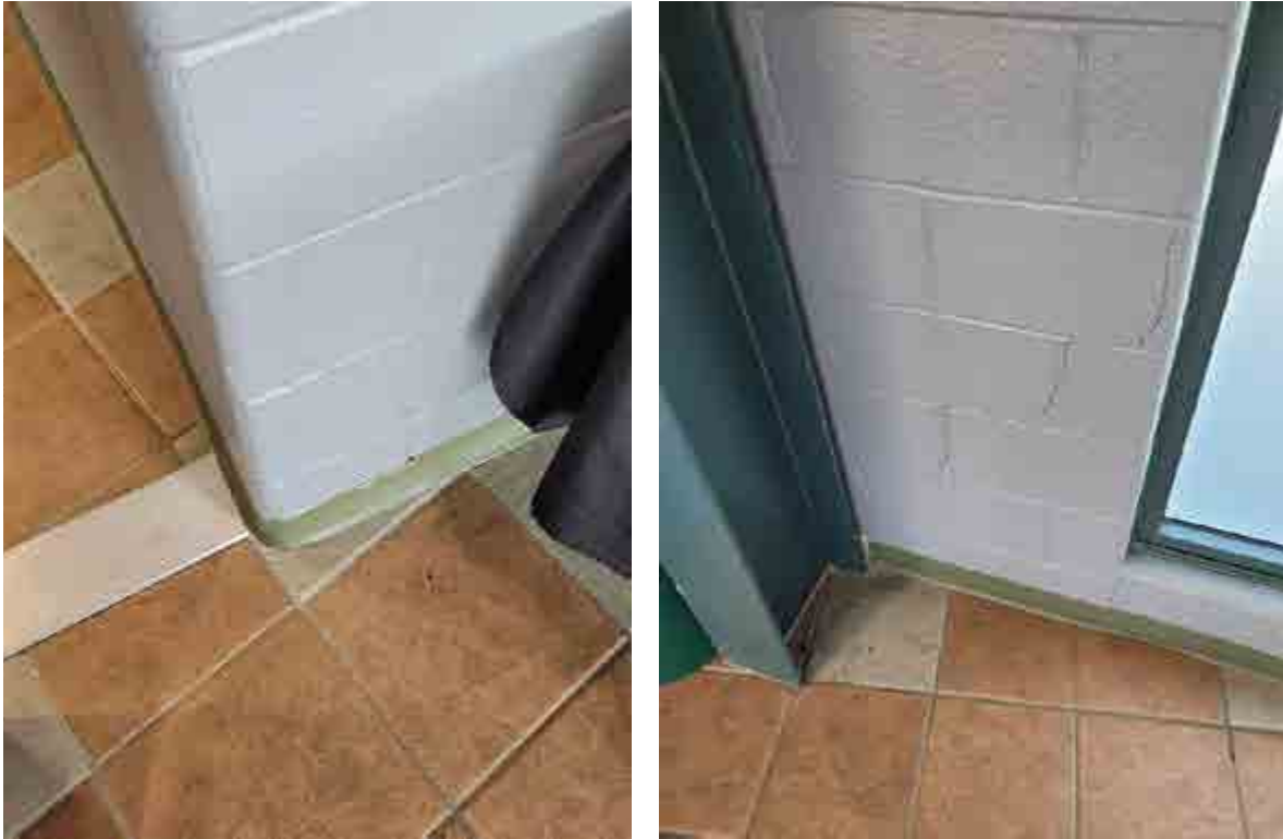
Cracking in CMU walls at Suite Level.
