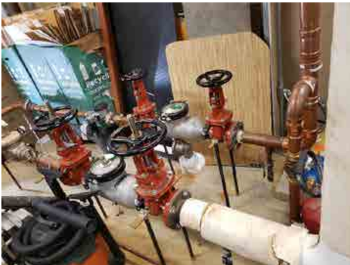
3" domestic water and 2 1/2" irrigation water meters and backflow preventers
