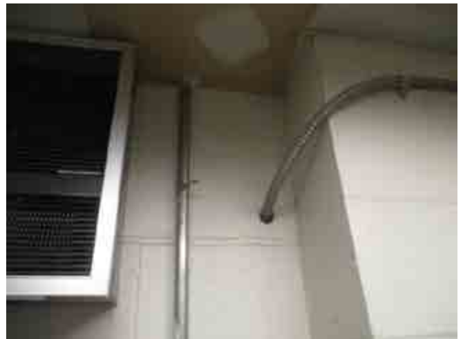
4. Relocate flexible conduit entering elevator #2 machine room
