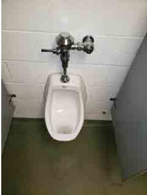
Manual flush valve Urinal and Water Closet at Home Team Clubhouse
