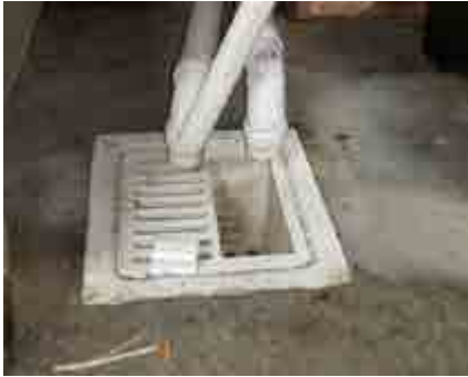
Floor sinks with grates and domes
