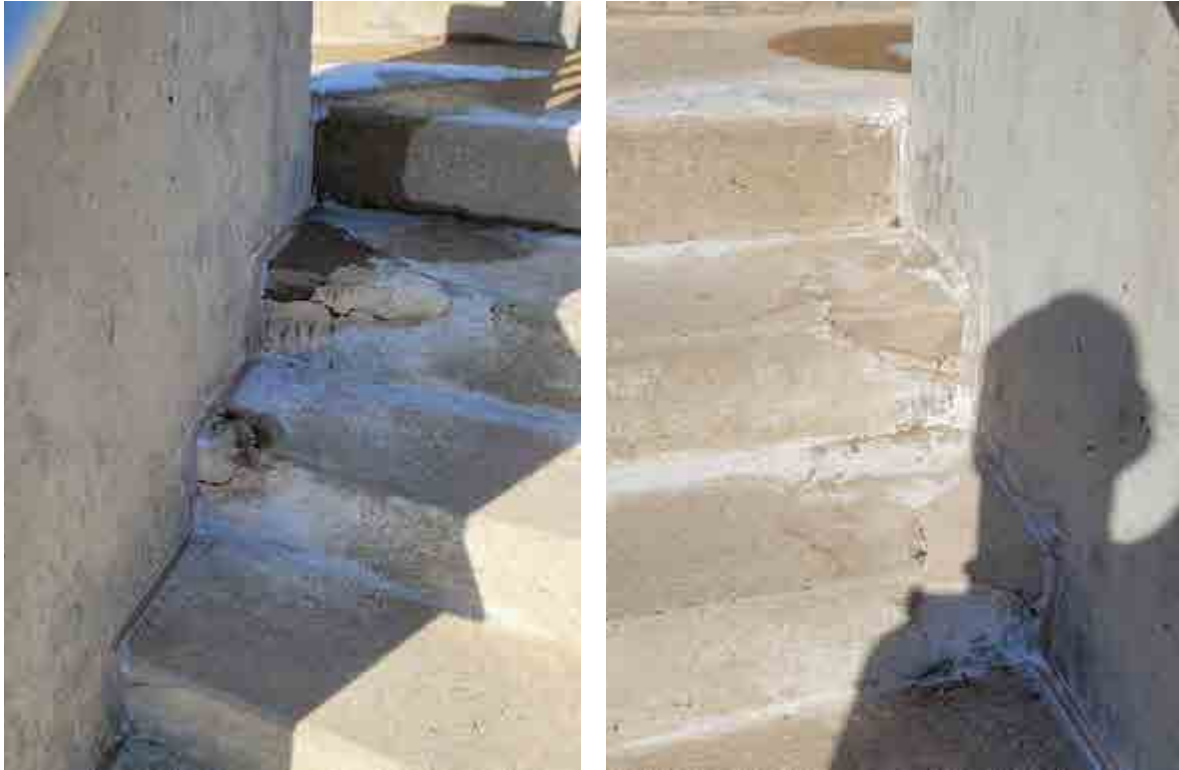
Spalls and cracking in CIP concrete cross aisle stairs.
