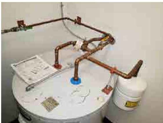
An electric 50-gallon water heater serves the Suite Bar.
