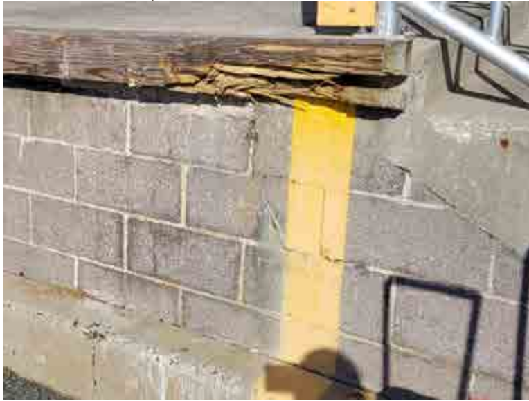
Damaged CMU wall at loading dock.
