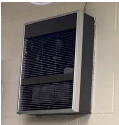
(17) Southern Eatery Electric Unit Heater (UH-X)
