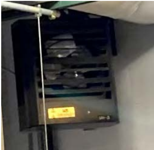
(20) Mechanical/Electrical Room Unit Heater (UH-3)
