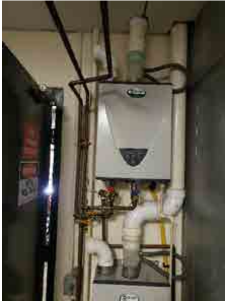
(2) Gas fired tankless water heaters serve the Commissary.
