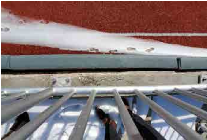
ASB-8 Cracking at sloped retaining wall
