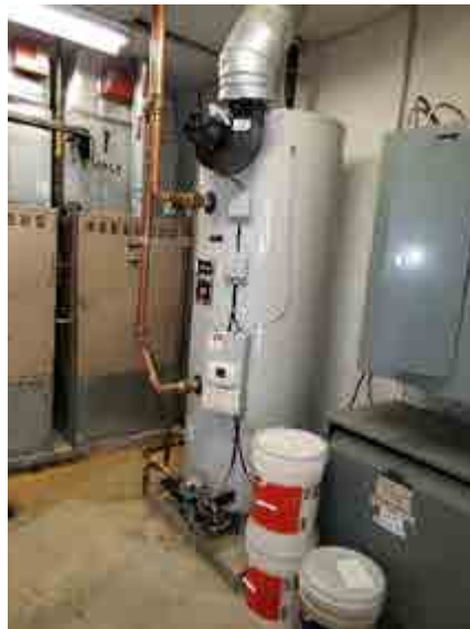
A gas fired 80-gallon storage tank type serves the Home Clubhouse
