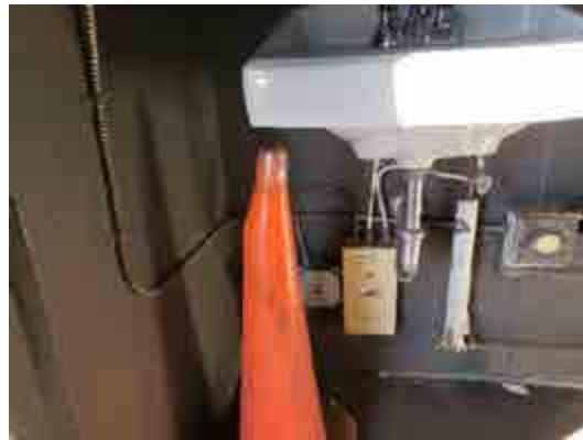
Electric Point of Use water heaters serve each Dugout
