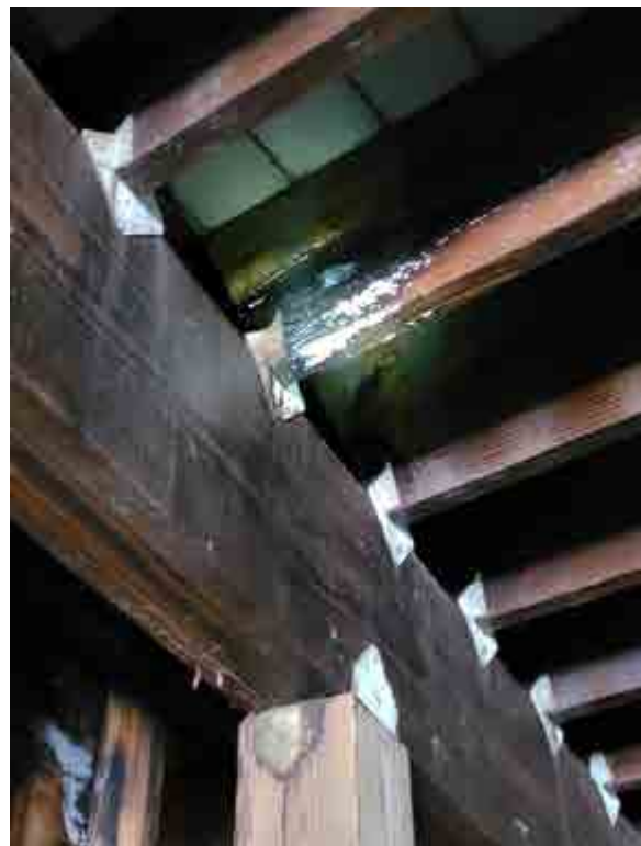
Deterioration of left field deck wood structure and connections.
