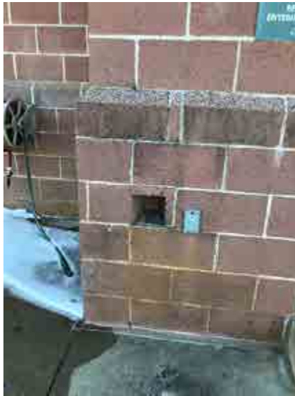
AHCE-3 Masonry Infill
