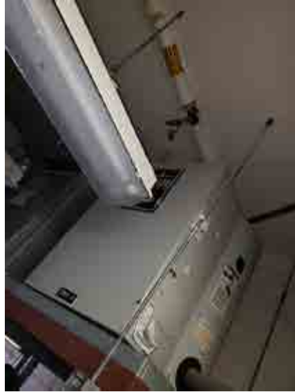
An electric 20-gallon water heater serves the Picnic Bar.
