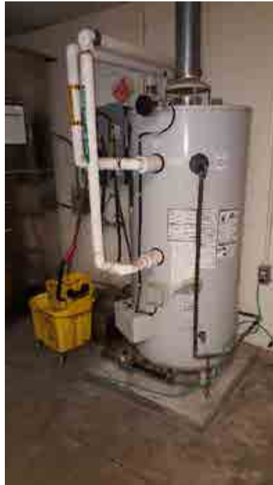
A gas fired 75-gallon storage tank type serves the North Concessions.
