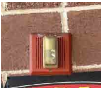
Corroded fire alarm outdoor strobes/speakers
