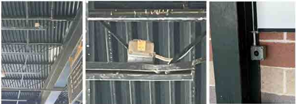
Exterior receptacles without coverings
