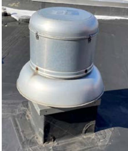
(19) Mechanical/Electrical Room Exhaust Fan (EF-10)
