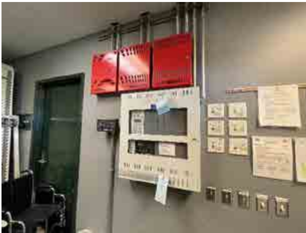
Existing Fire Alarm Control Panel
