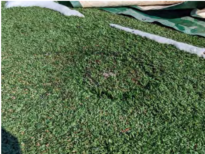
QUICK COUPLER BEHIND HOME PLATE – THE VALVE BOX IS INSTALLED TOO LOW WHICH CAUSES AN UNEVEN SURFACE.
