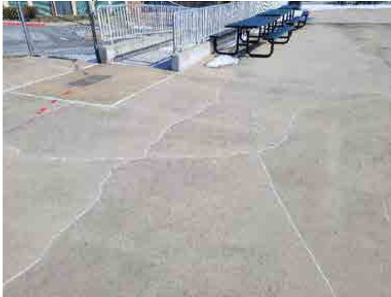
Cracked and settled left field concrete slab on grade.
