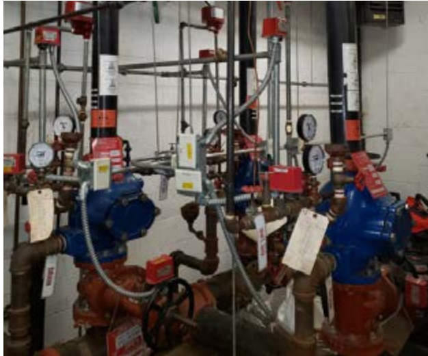
Dry Sprinkler Valve Assemblies
