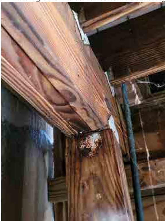
Deterioration of left field deck wood structure and connections.
