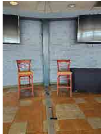
ASCI-32 Expansion joint covers
