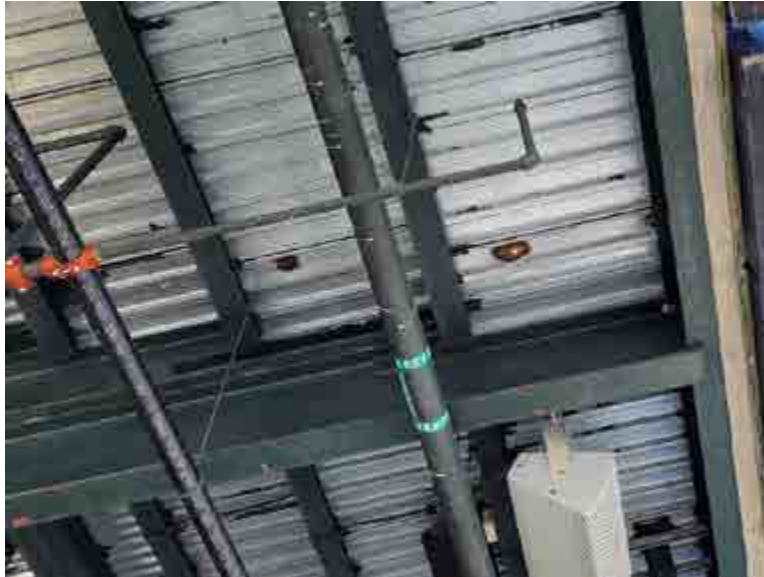
Corroded decking below suite level seating.
