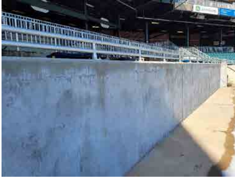
Cracking in existing parge coating on cross aisle wall.
