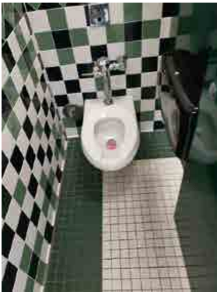
Typical hard-wired to manual flush valve replacement at water closets and urinals.
