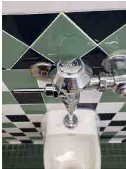
Typical hard-wired to manual flush valve replacement at water closets and urinals.
