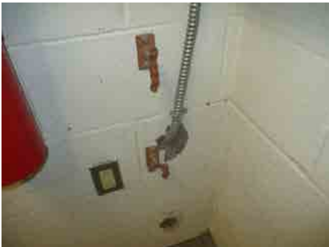
3. Relocate flexible conduit entering elevator #2 machine room
