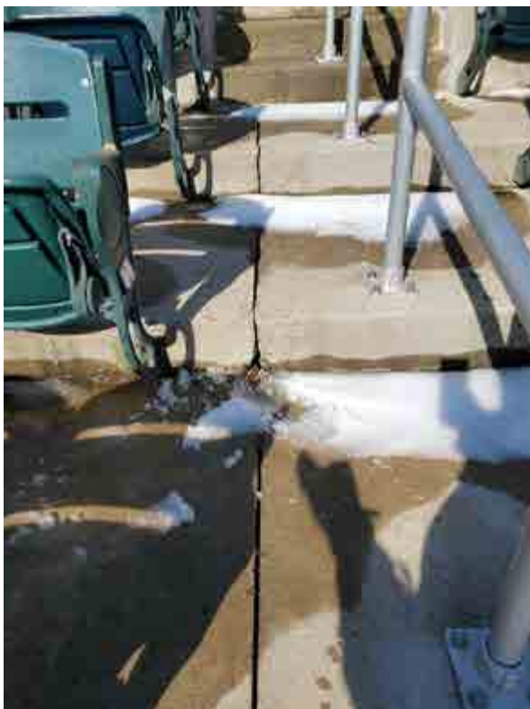
ASB-4 CIP control joints
