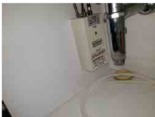
(12) Electric Point of Use water heaters are located below each lavatory and countertop sink to serve the Suites.
