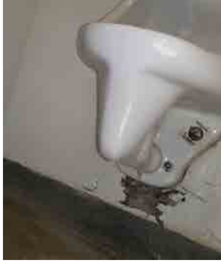
Water damage at Umpire Urinal
