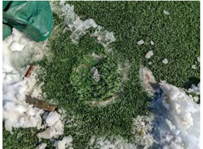
QUICK COUPLER BEHIND PITCHERS MOUND – NEED TO REPLACE BROKEN VALVE BOX LID.
