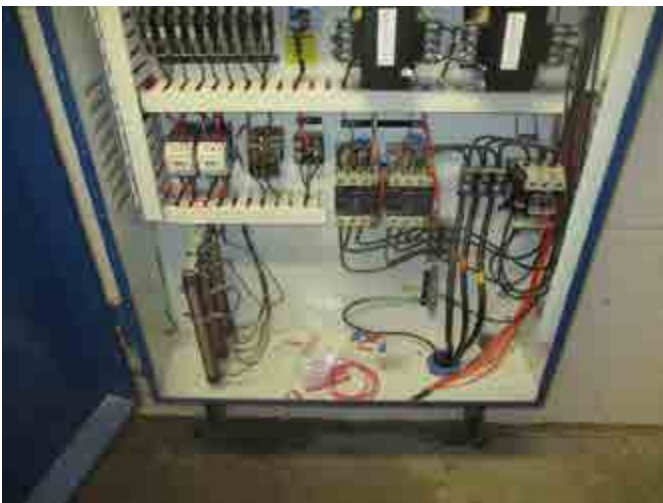
7. Clean out inside of controllers
