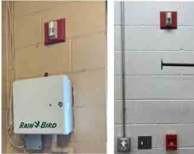
Outdated indoor fire alarm strobes/speakers
