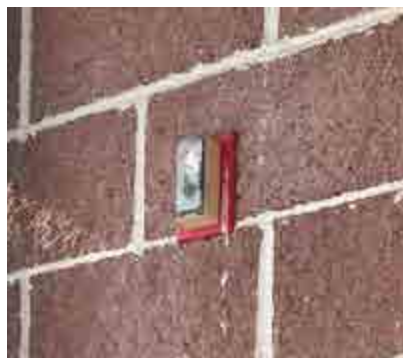
Corroded fire alarm outdoor strobes/speakers
