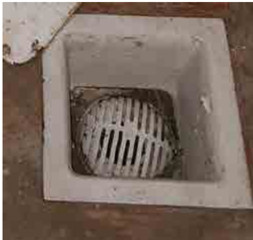
Floor sink missing strainer dome and a floor sink with the dome but no top grate
