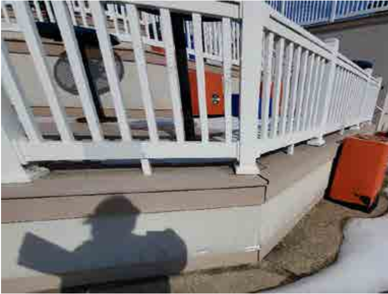
Damaged PVC railings at left field deck.
