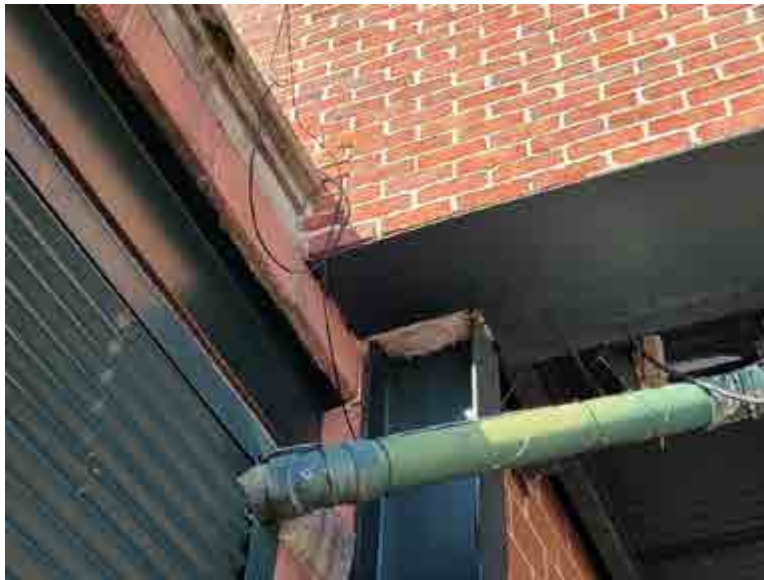
Deflected Brick Shelf and Cracking in Brick Veneer.
