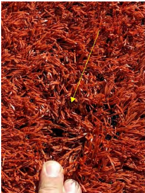
BASE ANCHOR HOLE FOR 60' BASES (YOUTH GAMES). TODD SAID PLUGS WITH TURF INFILL ON TOP ARE FABRICATED AND ARE INSTALLED FOR MiLB GAMES.
