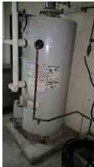
A gas fired 75-gallon storage tank type serves the South Concessions.
