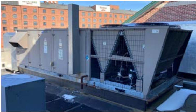
(2) Roof Top Air Handling Unit (RTU-5)
