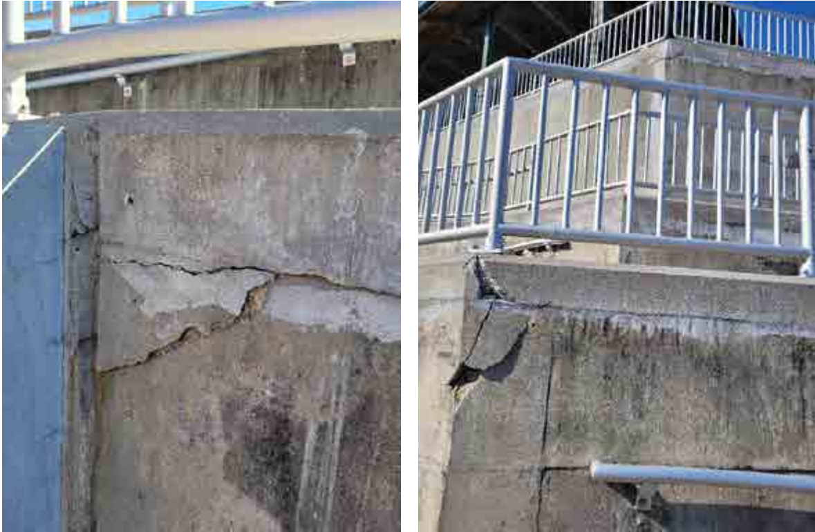
Spalls and cracking in CIP concrete walls at ramps.
