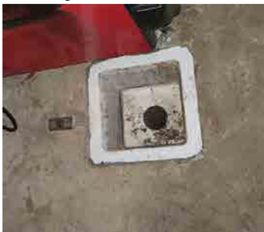
Floor sink missing strainer dome and a floor sink with the dome but no top grate
