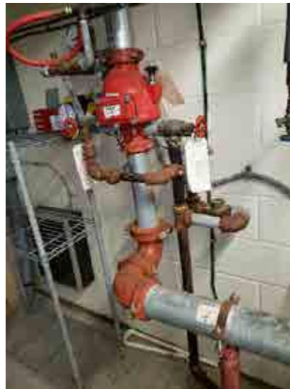
Dry Sprinkler Valve Assembly at Crab Shack
