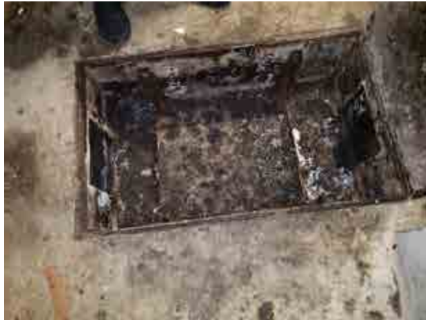
50 GPM Grease Interceptor below the stairs to serve each Concession
