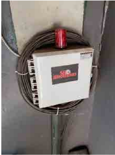
Team Dugout Sewage Ejector Pit and wall mounted Control Panel
