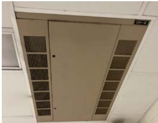
(16) Typical Gang Restroom Electric Unit Heater (UH-6)
