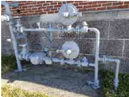
(2 PSI) Natural Gas Service Meter Assembly at Main Mechanical Room
