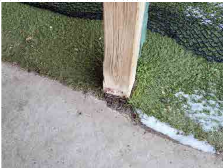
Corroded post bases at exterior 6x6 posts of clubhouses.
