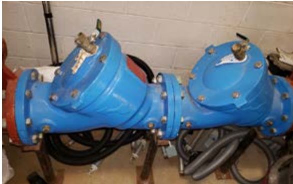
Incoming Fire Service Backflow Preventer at Main Mechanical Room
