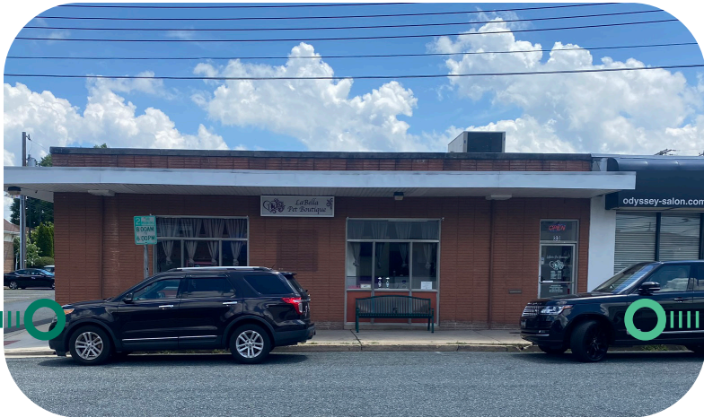
BEFORE: EXISTING CONDITIONS
