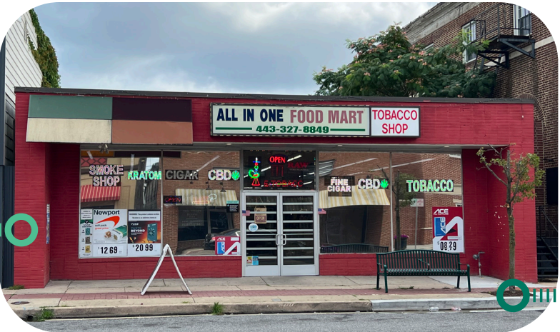
BEFORE: EXISTING CONDITIONS
