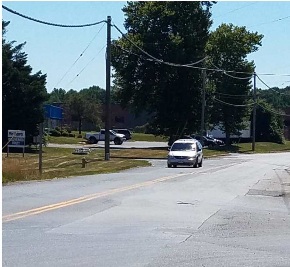
Old Philadelphia Road at MD 715 Looking West
