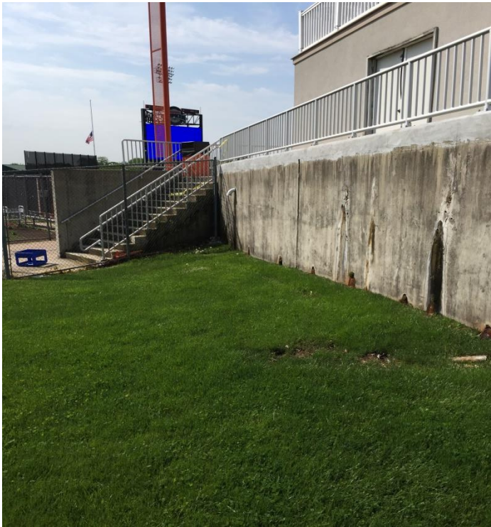
End of ramp at stair
