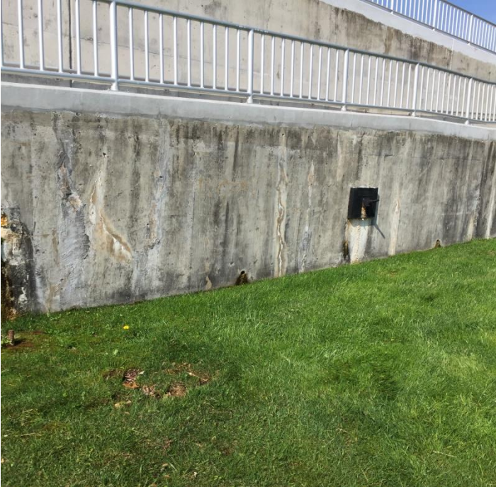
Pilaster and tieback anchor plate
