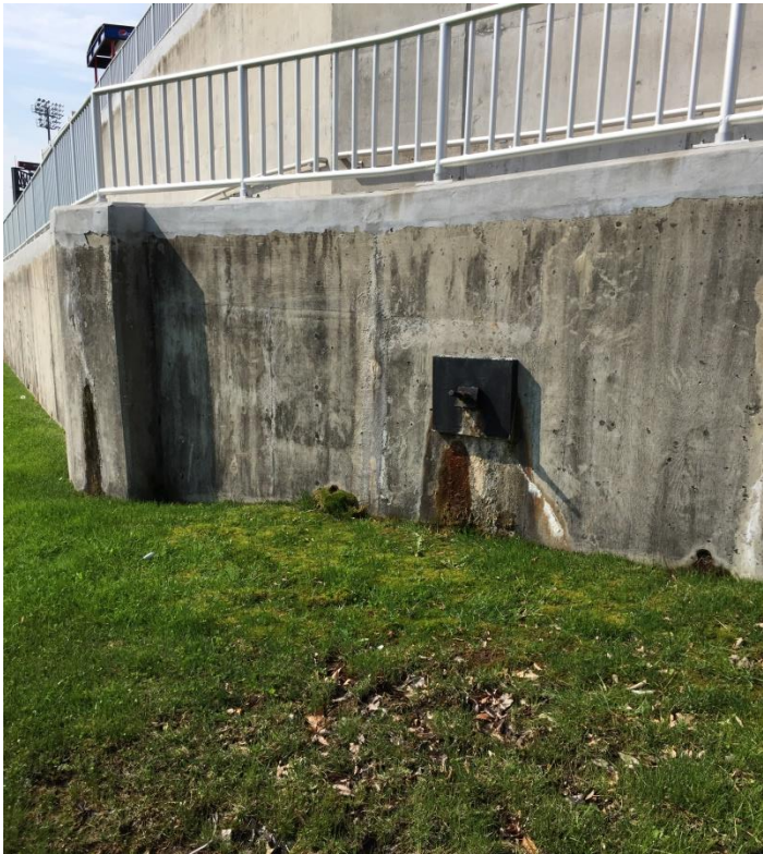
Pilaster and tieback anchor plate
