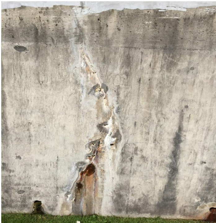
Previous crack repair by epoxy injection
