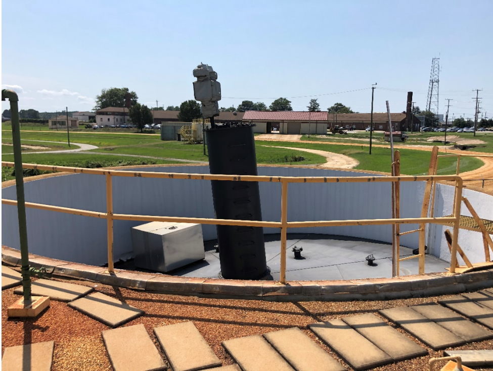
Top of Digester Building – Roof Elevation Looking at Digester #1
