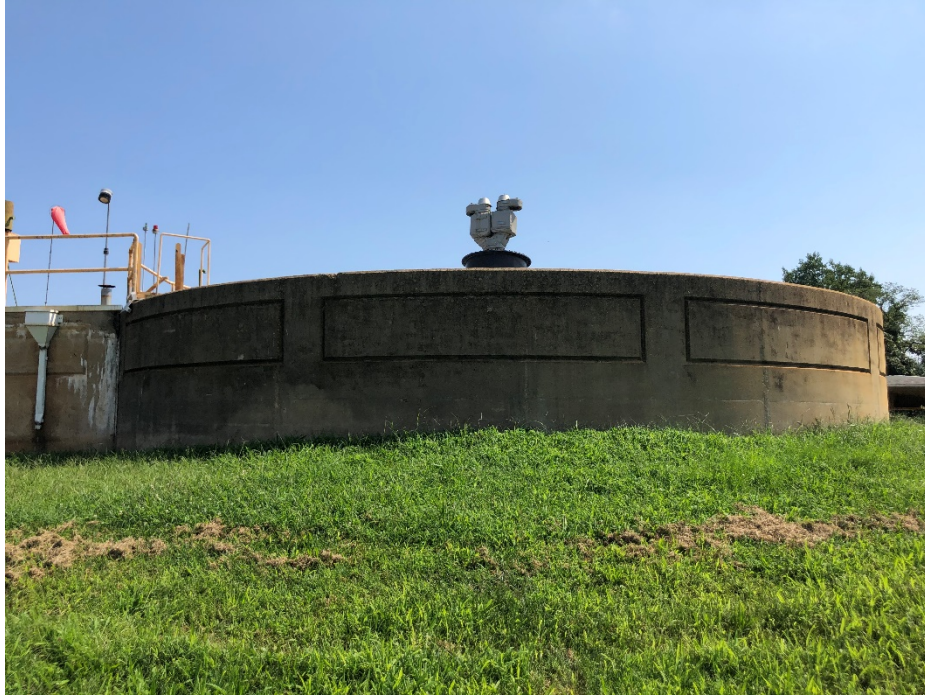
Digester #1 Tank Exterior – looking south
