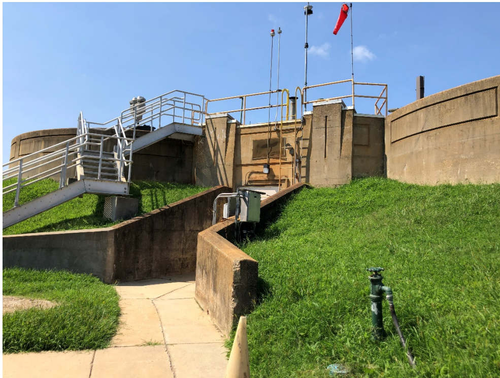
From Walkway to Digester Area – Digester #1 is on left
