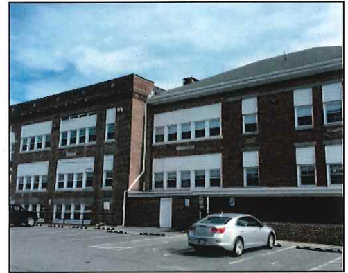
Clear Location of the Third Addition at the Central Core and South Wing
