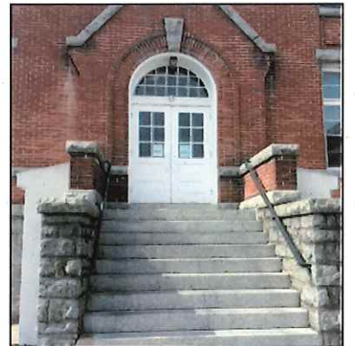
Exterior Stair at South Wing
