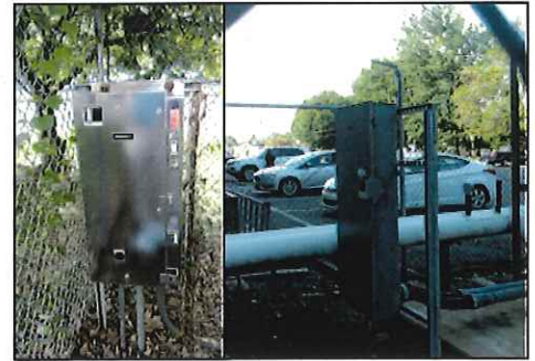
HVAC Equipment Disconnects
