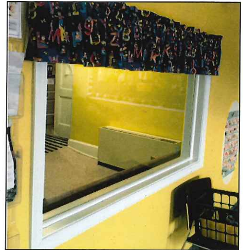
Framed Interior Window
