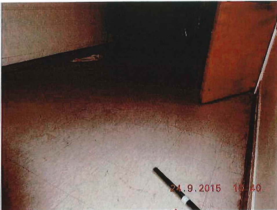
Photo 9 Non-asbestos 12" floor tile.
