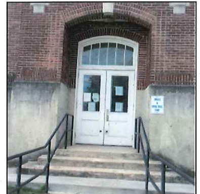
Exterior Stair at North Wing
