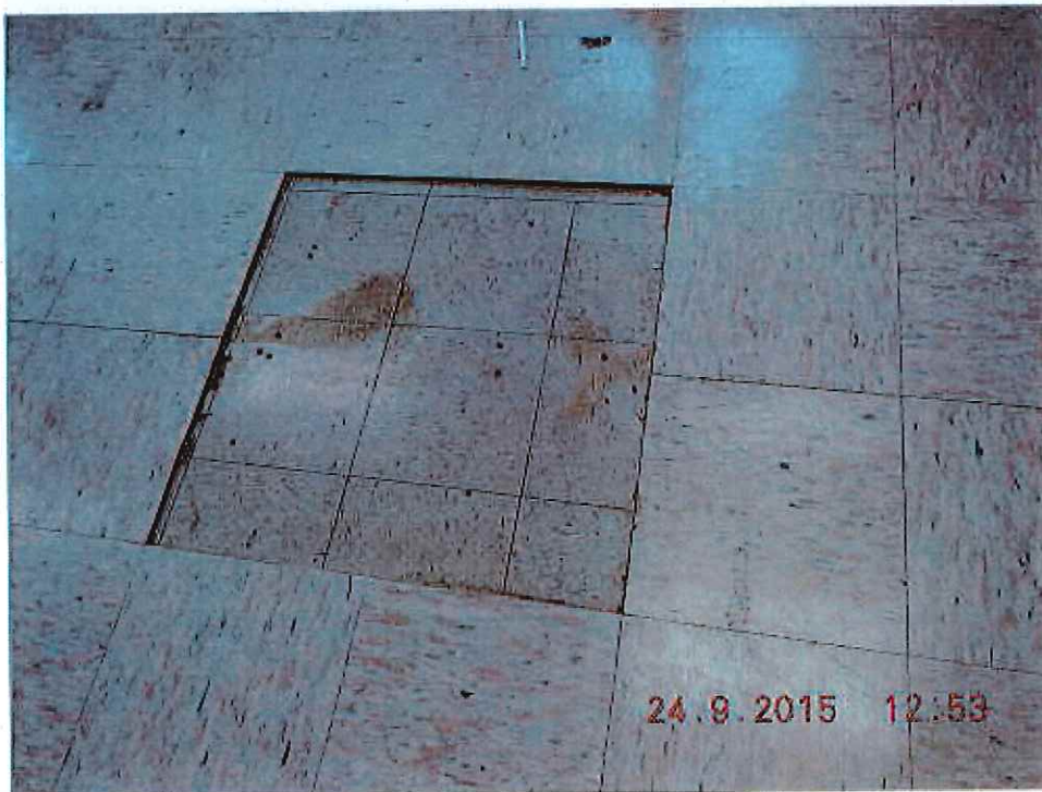
Photo 14 Typical with 12" VCT covering 9" VAT
