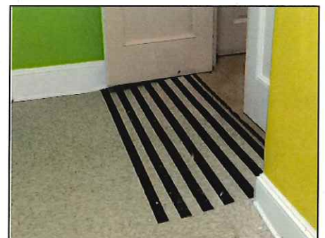
Interior Ramp at 3rd Floor into South Wing
