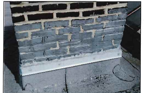
Repaired Flashing and Jointing
