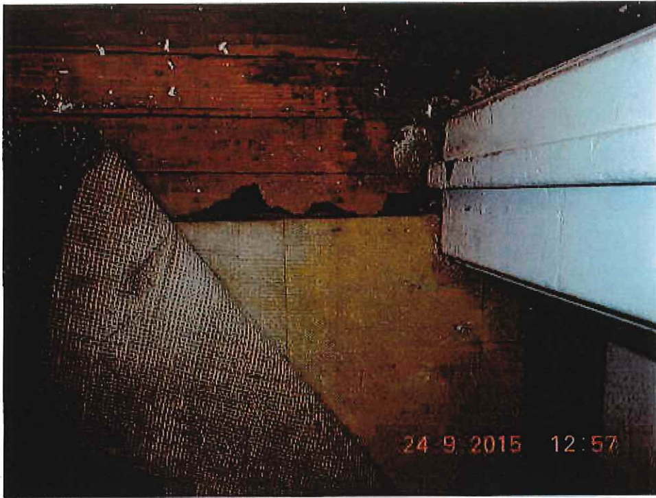
Photo 15 Typical with carpet covering 9" VAT
