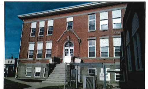
Downspout at Southwest Corner
