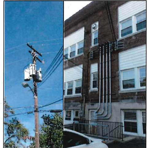
Pole Mounted Transformers and Conduit Running into Building
