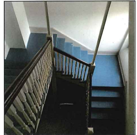
South Exit Stair
