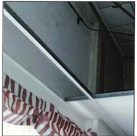
Lowered Original Window Openings from Inside
