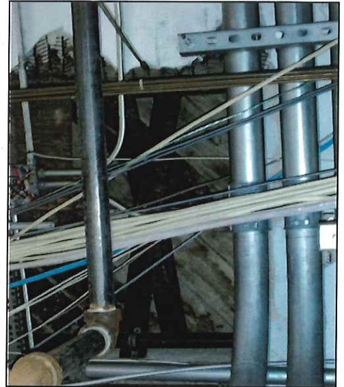
Opening in Ceiling Showing the Exposed Wood Plank Flooring
