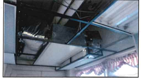
Two-Pipe Fan Coil System
