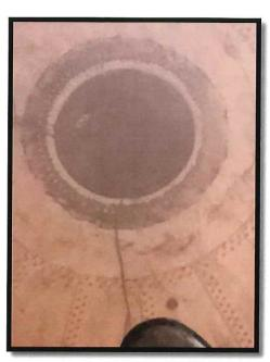
View of the interior roof and left behind spider rods.
