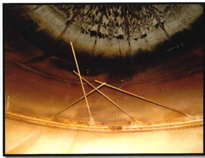
View of interior pictures post-washout showing remnants of cathodic protection system.
