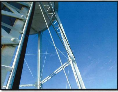
View of the access ladder, climb prevention plate, fall prevention cable, and cable stay.
