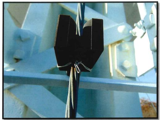
Pictured above is the cable stay where a wire has been implemented in order to prevent the fall prevention cable from pulling out.
